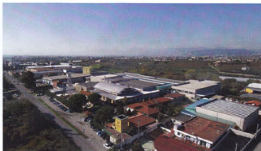
An aerial view of the Ovattificio Fortunato facilities
